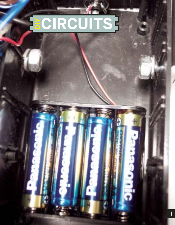
Fig. I: Interior of display panel unit with batteries, handle retaining nuts, and DIN connector jack.
