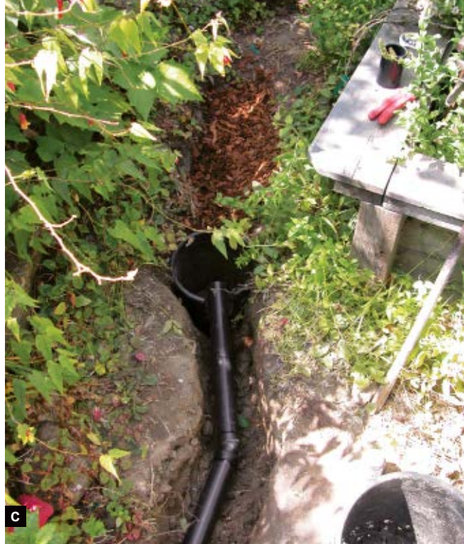
Fig. B: Pipes and pots for the double-ell split and right branch of the graywater system laid in the ground before burying. Fig. C: Left branch (with 16° elbow fitting) and irrigation terminal shown before burying.
