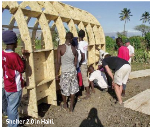
Shelter 2.0 built from construction lumber.
